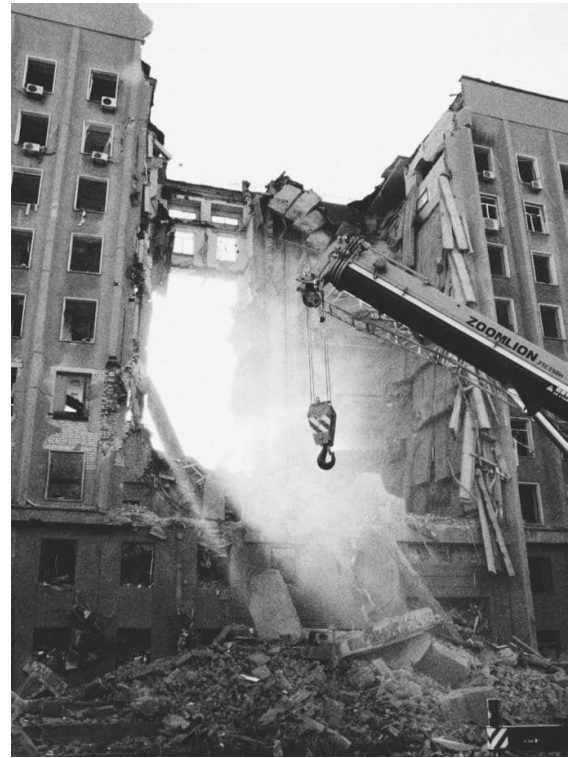
The building of the Commercial court of the Nikolaev area was destroyed by Russian bombs.
