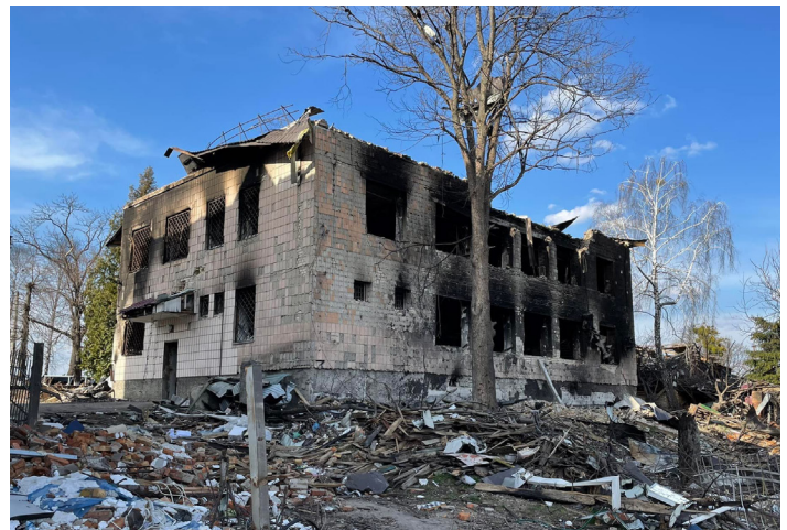
The building of the district court in Borodyanka was completely destroyed by Russian bombs.
